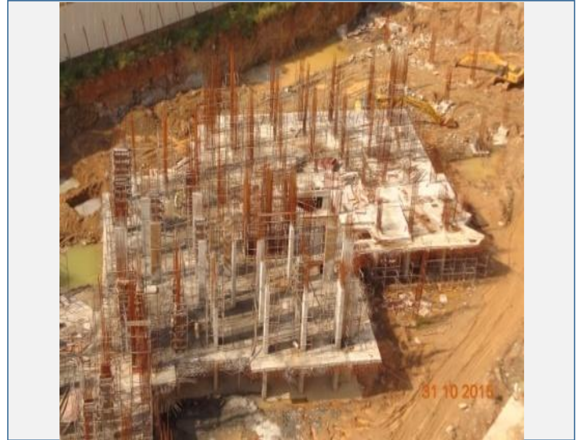
TOWER H : Upper Basement Column Casting Works in Progress.
