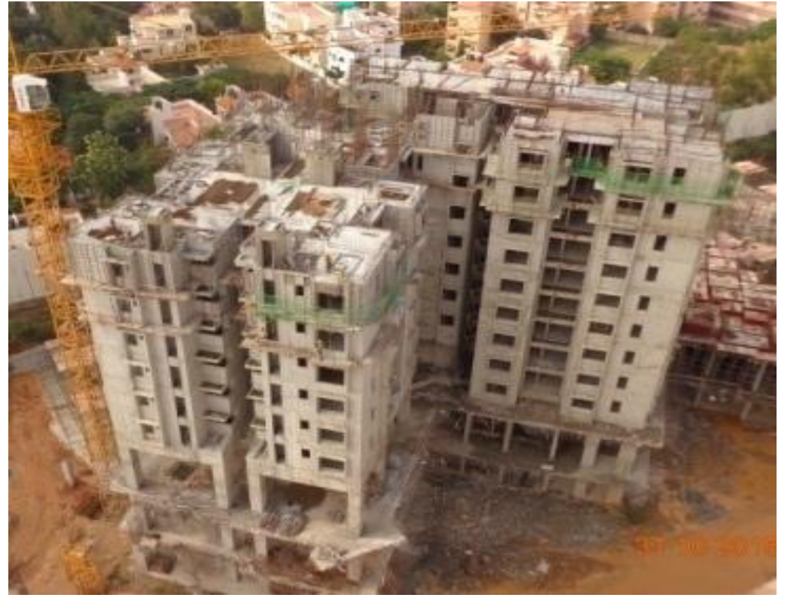
TOWER K : Level 9 Roof Shuttering & Reinforcement Works in Progress.
