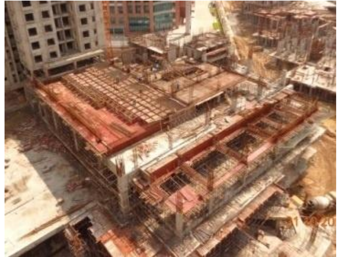
TOWER A : Level 4 Roof , Clubhouse Slab Reinforcement and Shuttering works in Progress.
