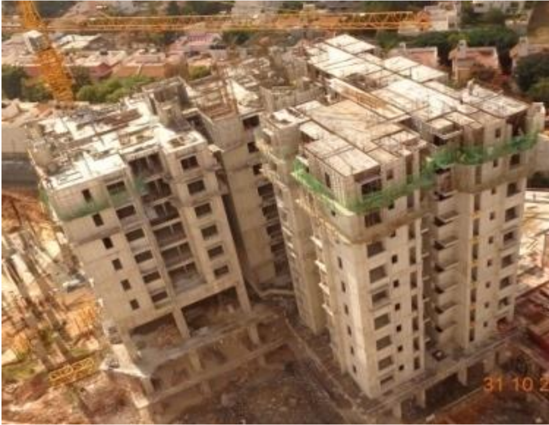
TOWER K : Level 9 Roof Shuttering & Reinforcement Works in Progress.
