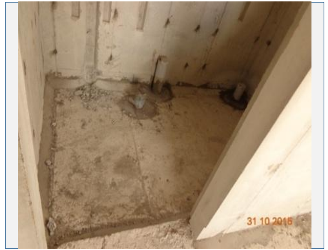
TOWER D : Terrace work and Toilet Bore Packing Works in Progress
