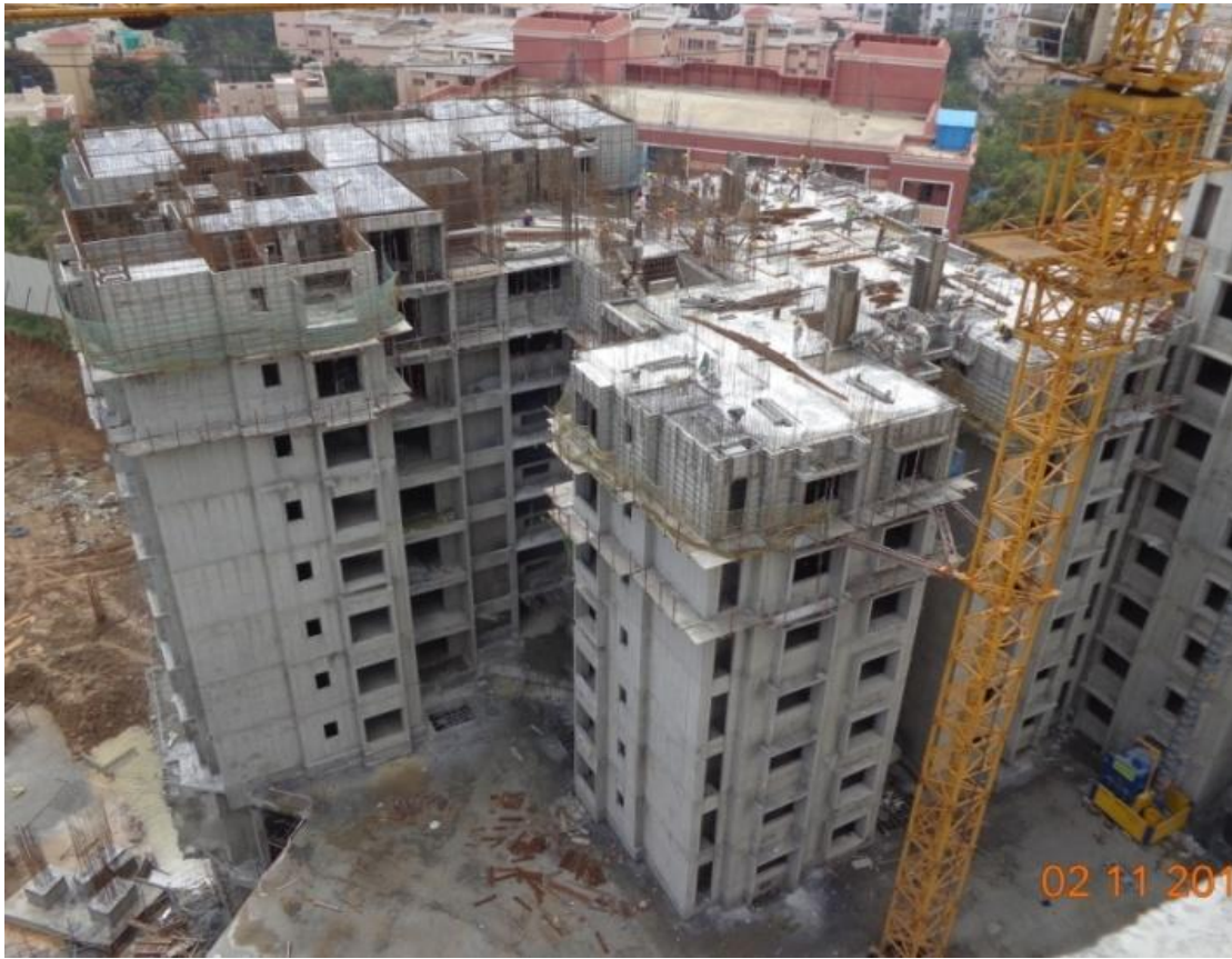
TOWER G : Level 8 Roof Reinforcement and Shuttering Works in Progress
