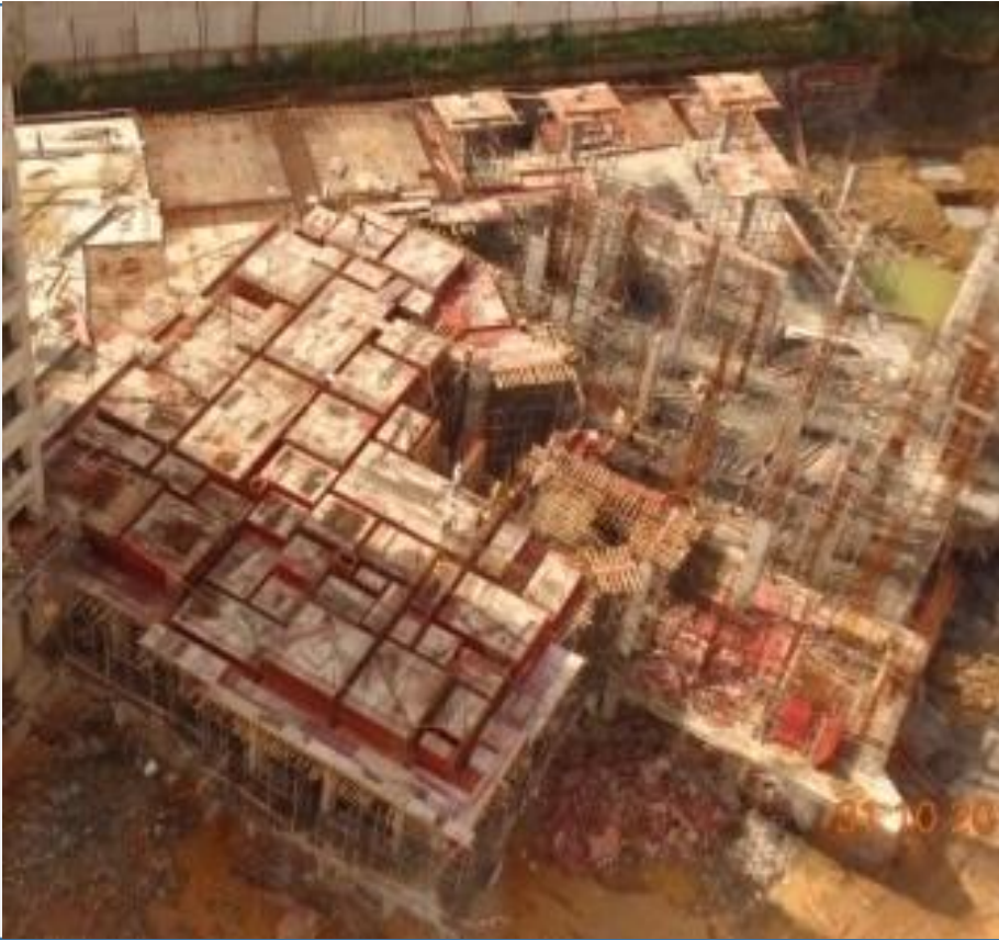
TOWER J : Upper Basement Column Casting , Slab Shuttering & Reinforcement Works in Progress .
