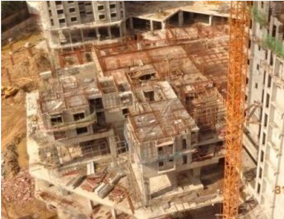
TOWER A : Level 4 Roof , Clubhouse Slab Reinforcement and Shuttering works in Progress.
