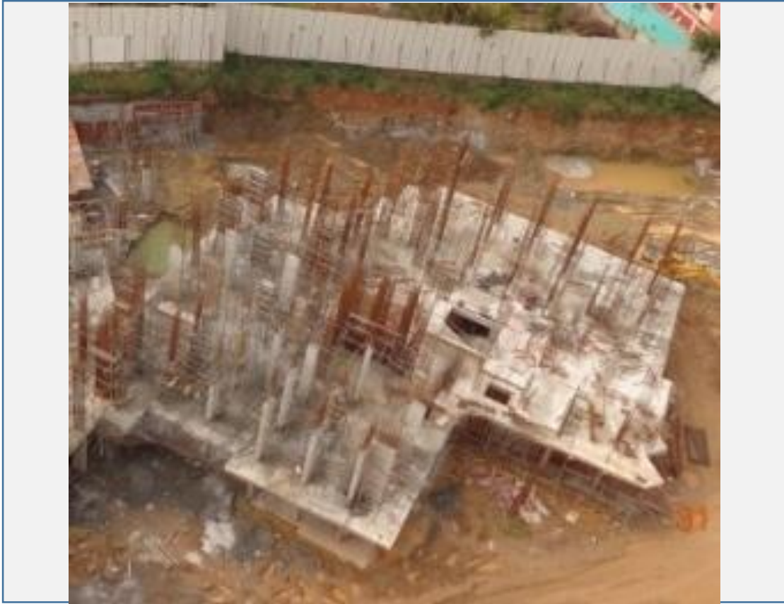
TOWER H : Upper Basement Column Casting Works in Progress.
