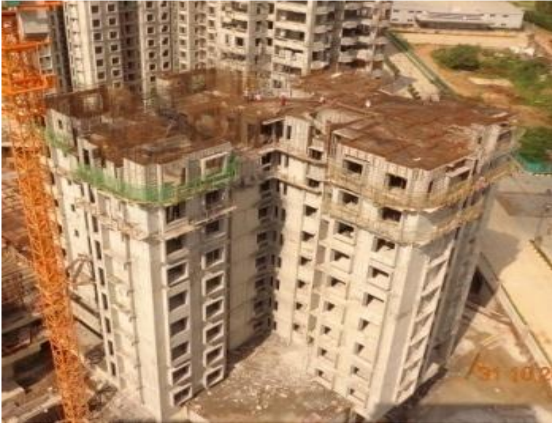
TOWER B : Level 11 Roof Shuttering and Reinforcement Works in Progress
